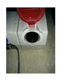
TAIL ADAPTOR MAY BE USED TO CONNECT TO 63AMP SOCKET AND GIVE 32AMP CONNECTION OR MAY BE DIRECT CONNECTION
