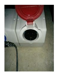
TAIL ADAPTOR MAY BE USED TO CONNECT TO 63AMP SOCKET AND GIVE 32AMP CONNECTION OR MAY BE DIRECT CONNECTION
