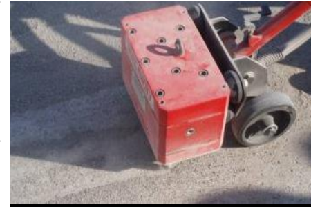
Laitance removal from concrete
