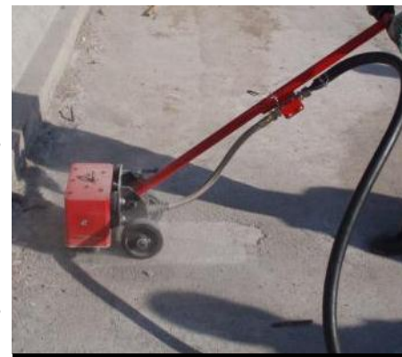
Scabbling bridge deck ready for sealant coating
