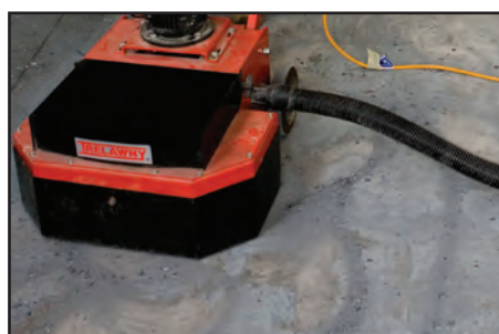
REMOVING HIGH SPOTS
